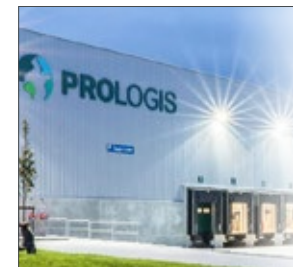
Prologis Southeast DC Distribution
